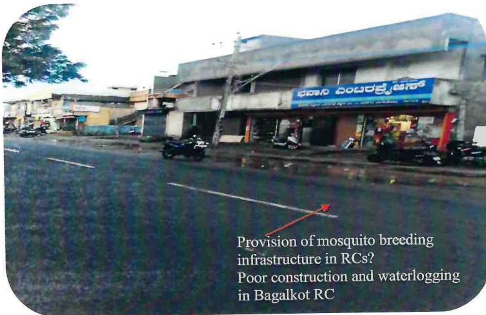
Picture A8.2:Poor Quality of Infrastructure in RCs
