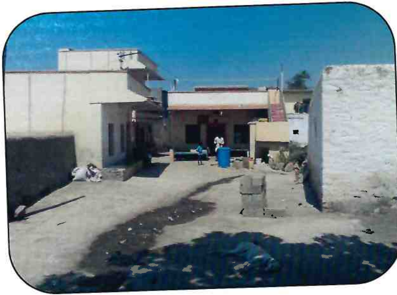
Picture A3.1: Poor Sanitation Facilities at Ankalgi Village
